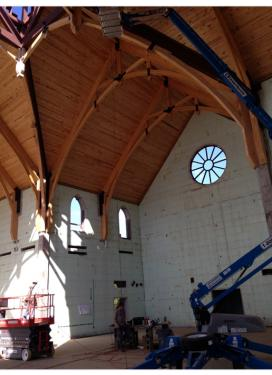
The project is the most complex use of ICF walls in and around the region. The complexity created by intersecting ICF wall thickness, arched openings, and the height of the unsupported gables pushed the limits of this type of construction.
