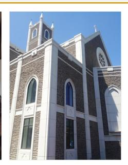
interior walls are built using ICF. St. Peter's was constructed with NUDURA's reinforced ICF walls with rebar and 2-way concrete slabs to floors. To emulate its English origins in style, the exterior is finished in cast stone and rock cast stone veneer.
