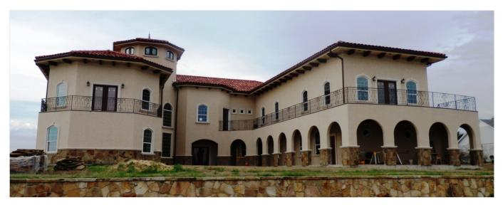
Each segment of the U-shaped home extends approximately 30m, long enough to cause concerns about floor deck shrinkage. Since an expansion or movement joint was undesirable, special consideration had to be given to floor cracking in the reentrant corners as well as ensuring that deck shrinkage did not cause excess irregularity to the walls.
